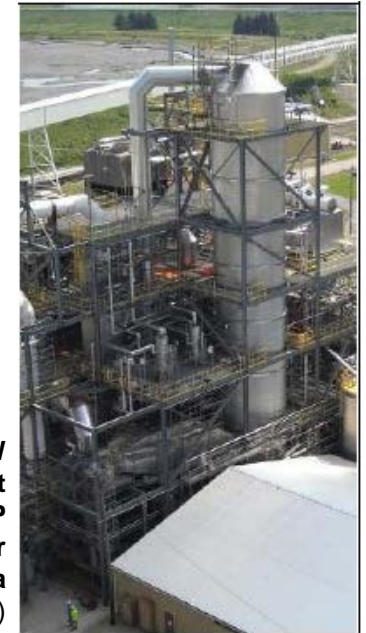
Alstom 20 MW Pilot Plant AEP Mountaineer West Virginia (USA)
