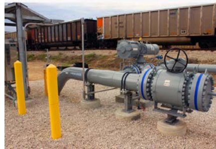
The CO 2 is used for EOR. Sent through this pipeline inlet at ~ 130 bar
