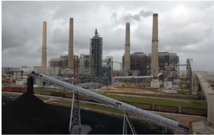
The Petra Nova 240 MWe carbon capture project at the WA Parish generating station, NRG Energy, southwest of Houston, Texas
