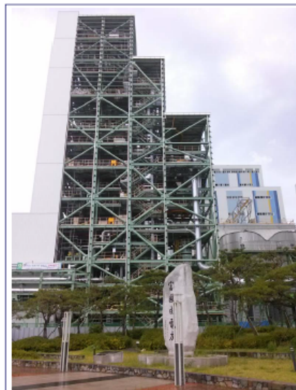
10 MW Pilot Plant at KOSPO's Hadong coal-fired power plant, Unit # 8
