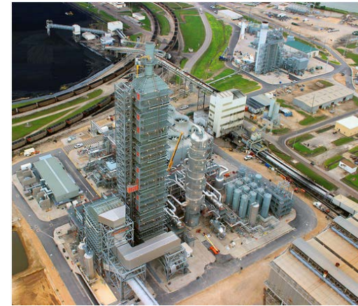
Carbon capture facility. Absorber Tower in the foreground. Regenerator Tower next to it . Co-generation system at the top right
